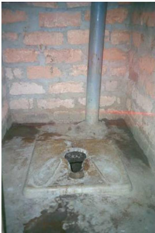
**Figure 7:** The ventilation pipe could be inside or outside depending on choice. The critical technical specification being the height of the pipe above the pit and the way the pipe faced the prevailing winds. (Photo provided by Paul Deverill, WEDC).
