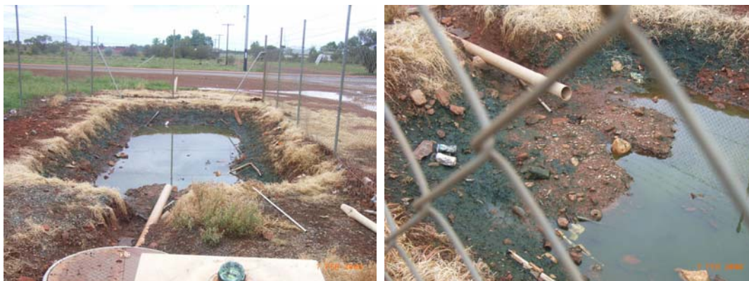
Figure 2: Inlet pipes and beer can from overflow sewerage treatment ponds (photo from Bill Atyeo, Environmental Health Officer, Wiluna).
