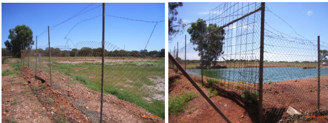
Figure 5: Fence Breeches sewerage treatment ponds (photos from Bill Atyeo, Environmental Health Officer, Wiluna).
