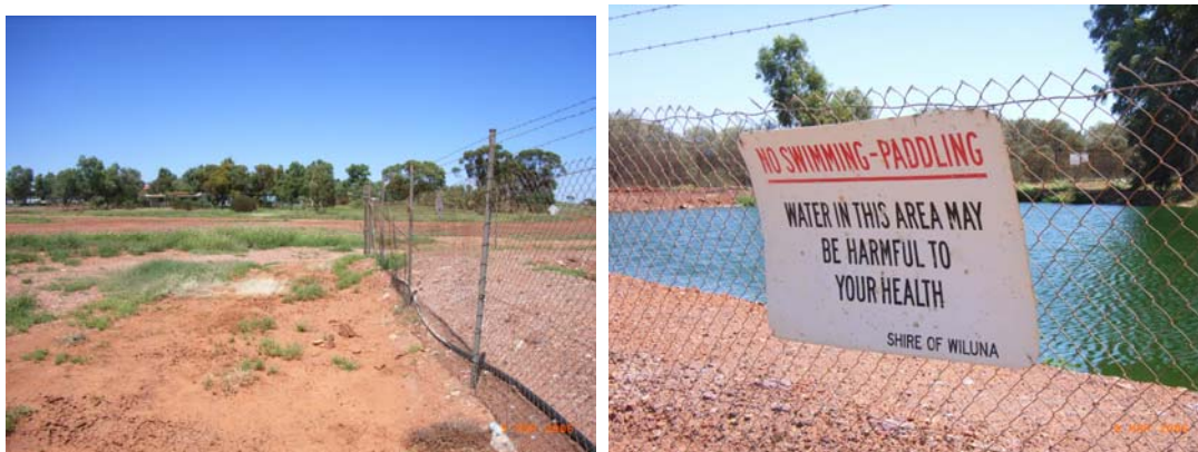
Figure 4: Overflow area top photo, sewerage treatment ponds (photos from Bill Atyeo, Environmental Health Officer, Wiluna).
