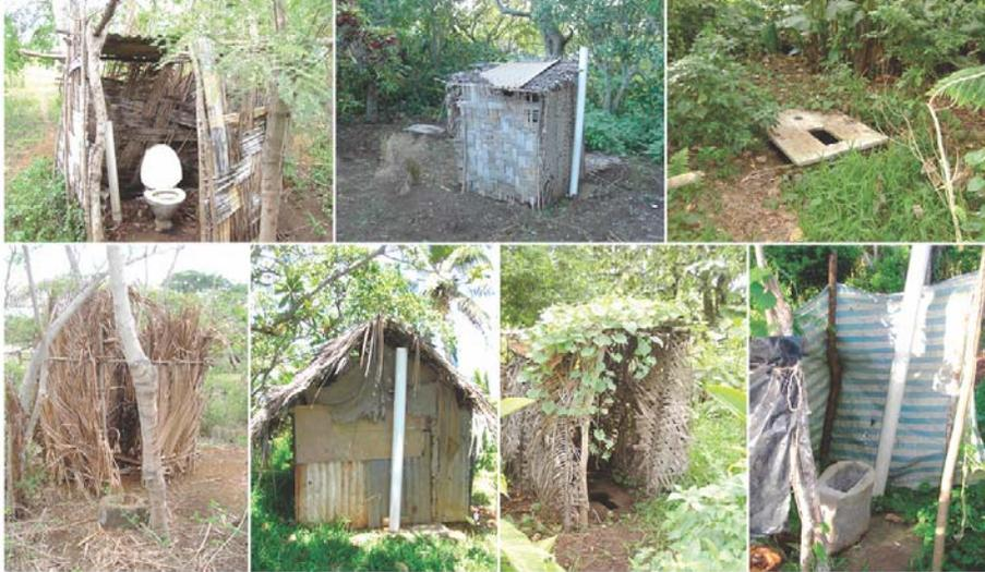
**Figure 4:** Examples of poorly constructed and maintained VIP latrines on Tanna Island.
